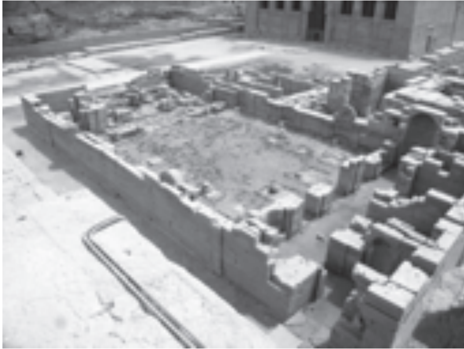
Figure 1. The basilica of Dendara seen from the roof of the Roman mammisi . © Ramez Boutros.
